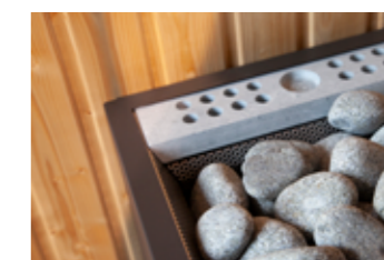
Detailed view of evaporator
